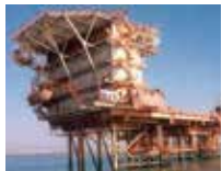
ENIMED - Gela 1 Platform: ECOMar 70 STP System - ATEX
