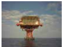
ENIMED - Perla Platform: ECOMar 70 STP System - ATEX
