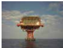
ENIMED - Perla Platform: ECOMar 70 STP System - ATEX
