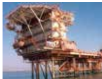
ENIMED - Gela 1 Platform: ECOMar 70 STP System - ATEX
