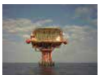
ENIMED - Perla Platform: ECOMar 70 STP System - ATEX
