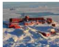
CHILEAN NAVY - Antartic base Punta Arenas: ECOMar 145 STP System
