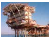
ENIMED - Gela 1 Platform: ECOMar 70 STP System - ATEX
