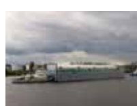
ZELENODOLSK SHIPYARD - Floating dock: ECOMar 24 STP System
