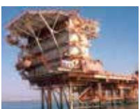
ENIMED - Gela 1 Platform: ECOMar 70 STP System - ATEX
