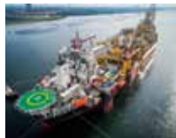
SAIPEM - Kaombo FPSO: Potable water treatment
